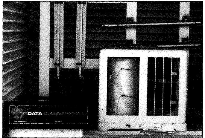
Temperature recording with the use of a pengraph.
